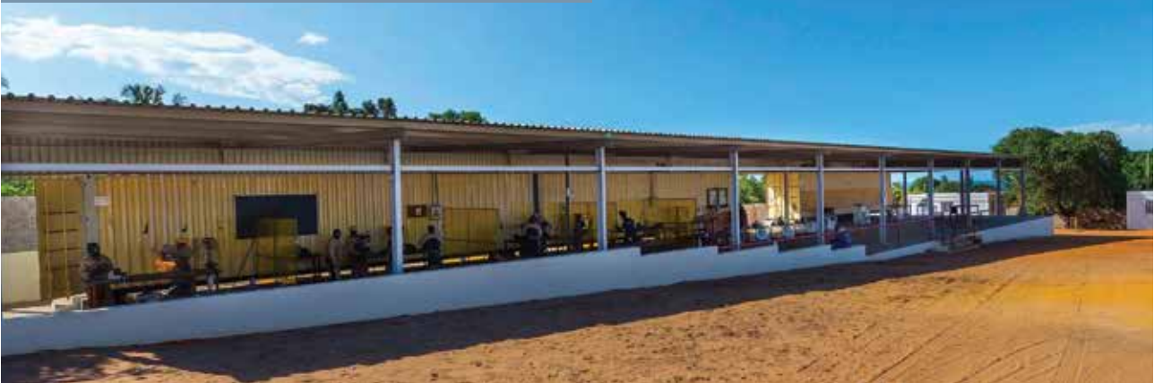
Training centre in Inhassoro, Inhambane Province, Mozambique
